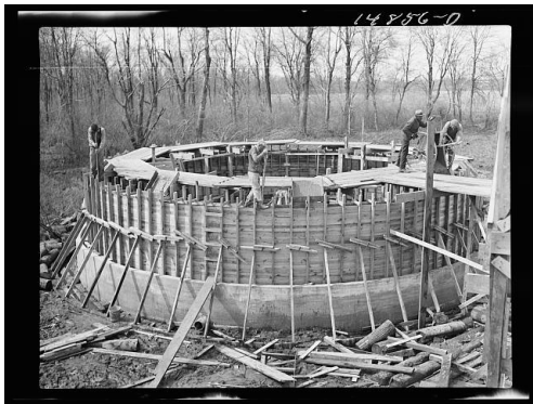
Fig. 4.1: Construction of sewage treatment plant in 1936/7 xlv
