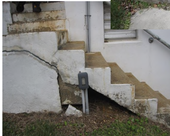
Deteriorated Concrete
