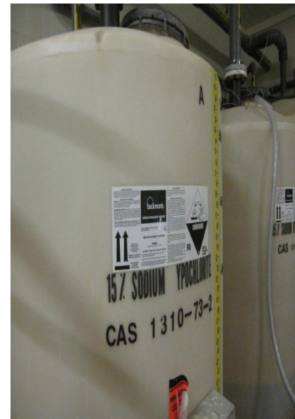
STP Sodium Hypochlorite Storage Tank
