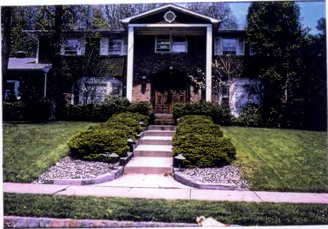
Elevated, Embellished House - imposing homes scored poorly.
